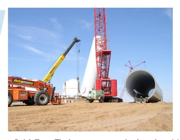
Quick Fact: The bottom tower section has a base 16-foot diameter and weighs 39 tons.
